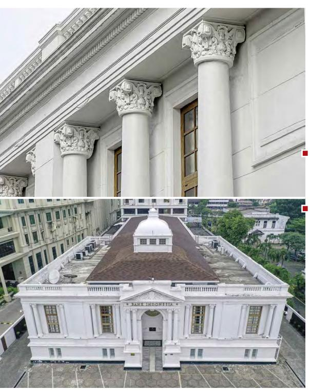
The additional roof on either side of the old building, uses a concrete deck. At the edge of the roof, there is also a parapet around the entire roof. The parapet is finished with balusters shaped like rows of flower vases.
