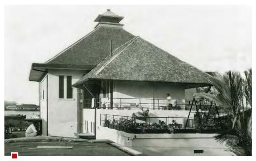
**Rear View |** This view at the back of De Javasche Bank Pontianak building showing the vault which is separate from the main building. The roof surface of the vault is coated with rainwater-retaining asphalt and covered with a small garden.
