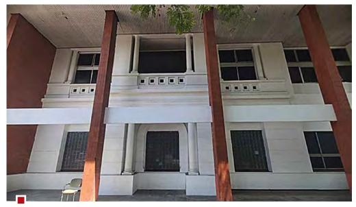
**Building Expansion |** The expansion of the building to the right and left sides meant that the old roof had to be demolished and replaced by a new, wider and longer roof. As a result, the front facade of the original De Javasche Bank building, which was preserved intentionally, was covered by the new roof extension.
